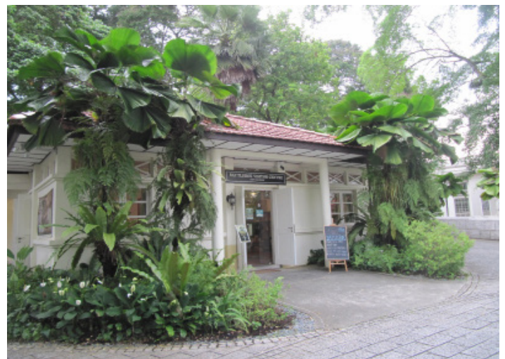
Figure 1: Battlebox Exterior. The Battlebox at Fort Canning: sealed up for 20 years, now a major tourism location.
